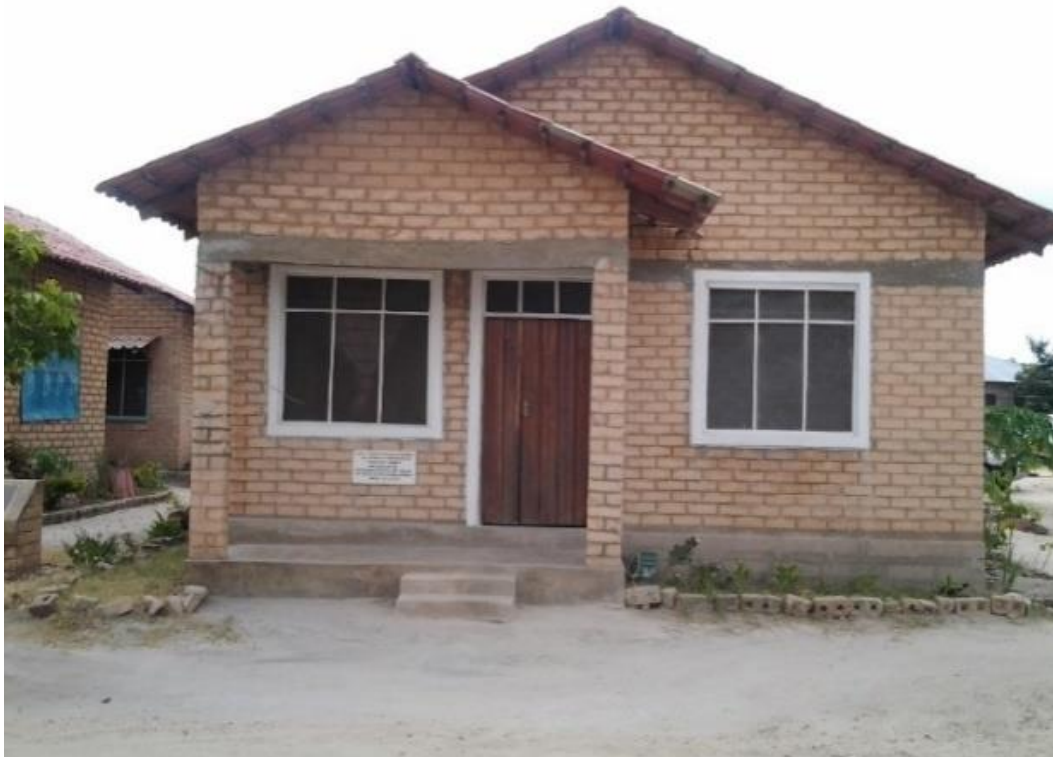
Muongano housing cooperative (Chamazi-Dar es salaam)
