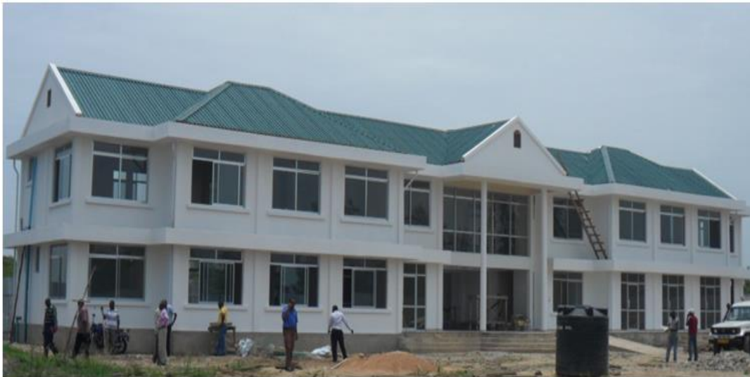
Jengo la Utawala la Sokoine Memorial High School-Mvomero lililosimamiwa na NHBRA
